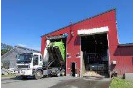
Shikao Biogas Plant
