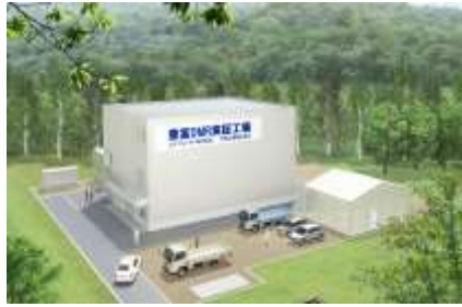
Hydrogen plant under construction
